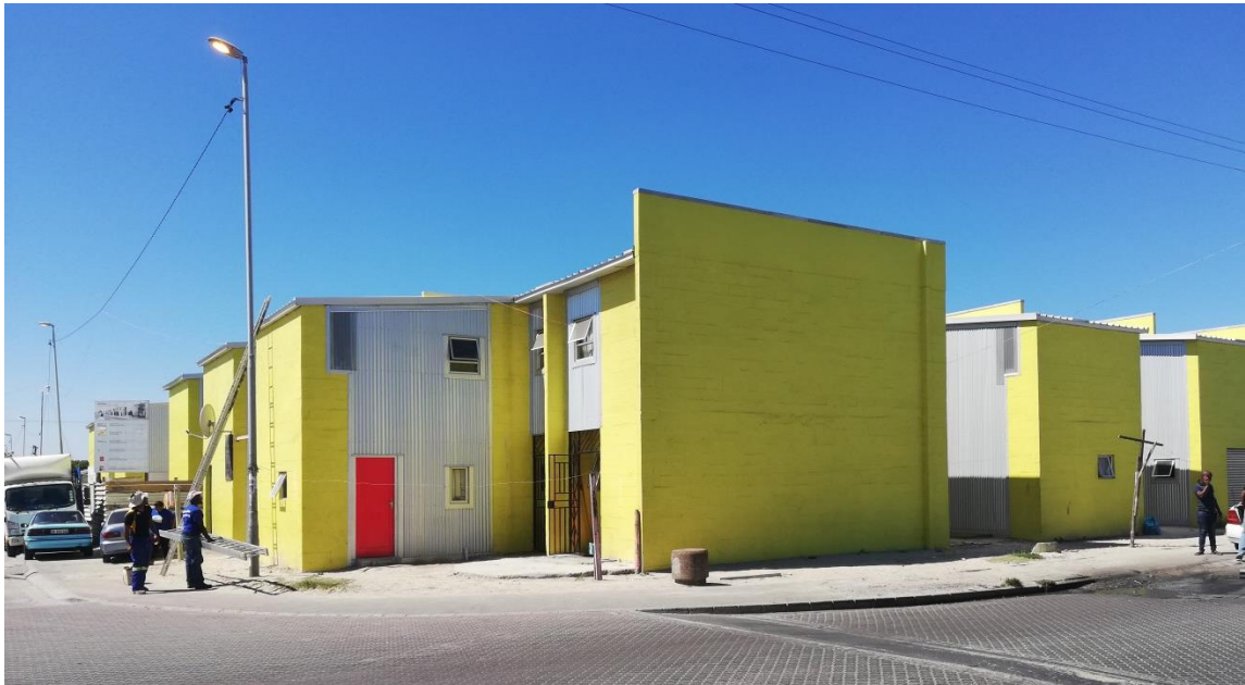
Photograph B3: BBT North Enhanced Reblocking
