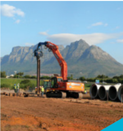
There are roughly 10 000 kilometres of water and sewer reticulation across Cape Town.
