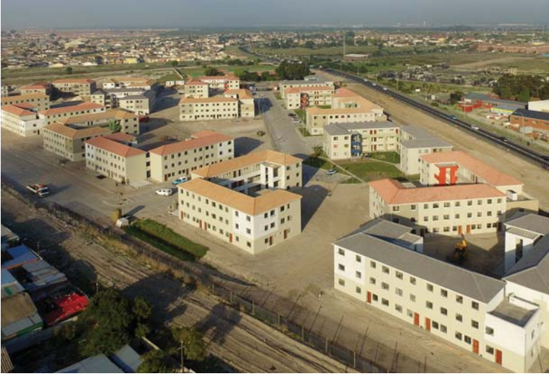
Two-time winner: The Belhar Gardens housing project offers 630 affordable units.
