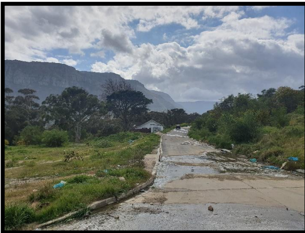
5. Onsite Street view from south to north showing existing infrastructure & site features.
