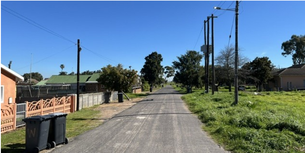
Existing residential erven along Main Road
