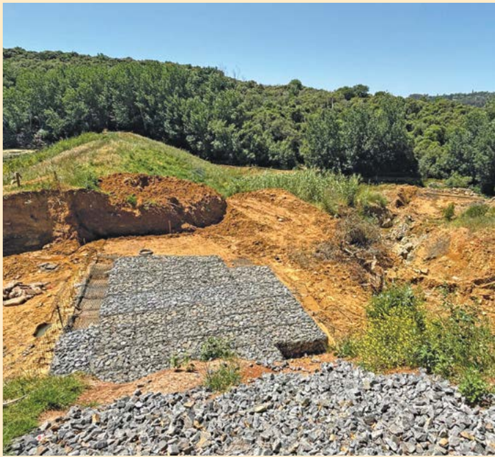
Helping the flow at Fynbos: The new spillway discharge channel being constructed at Majik Forest's Fynbos dam.
