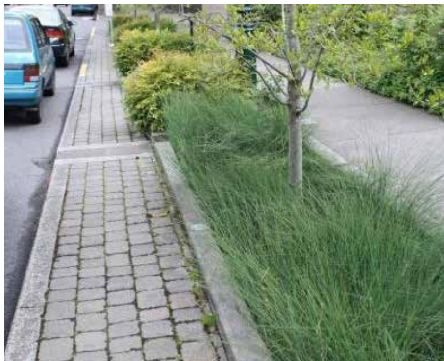
Fig. 6.29. Green street with swale
