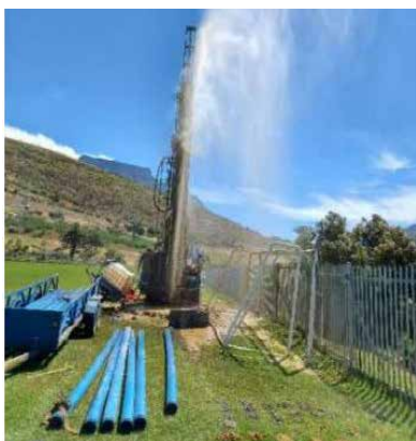
Fig. 4.101. Borehole Drilling at Target B (HHO, 2022)
