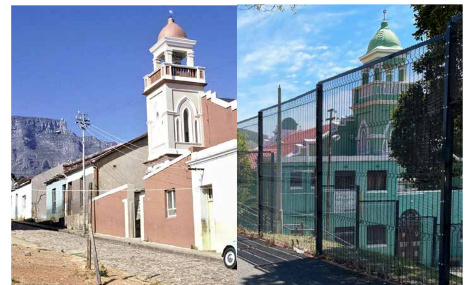
Fig. 3.26. A photo of Ellesmere Mosque from Ellesmere Street, dated 1973 Fig. 3.27. A present day view of Ellesmere Mosque from Constitution Street
