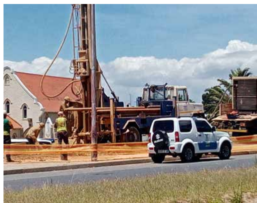
Fig. 4.100. Borehole Drilling at Target A (CCT, 2021)
