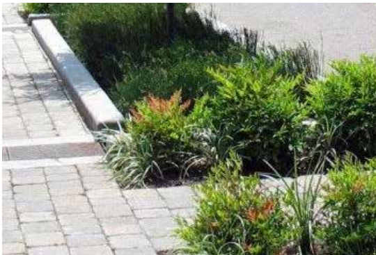
Fig. 4.110. Bio-Swales collect, treat and convey stormwater
