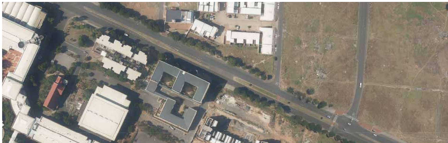
Fig. 5.116. Aerial photograph of New Hanover Street
