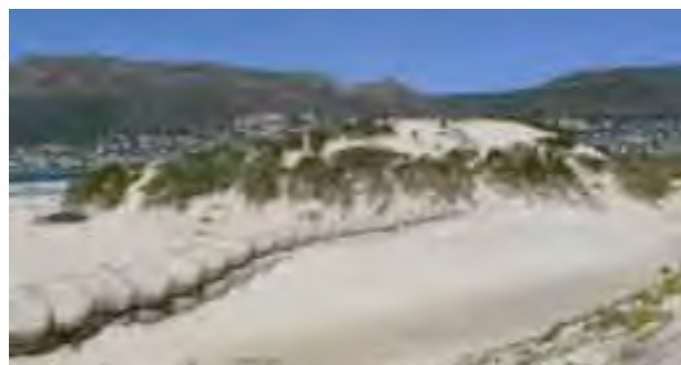
Sand bag type gabions are used to stabilise dunes at Clovelly. Wind-blown sand is a problem here as it affects the nearby railway.
