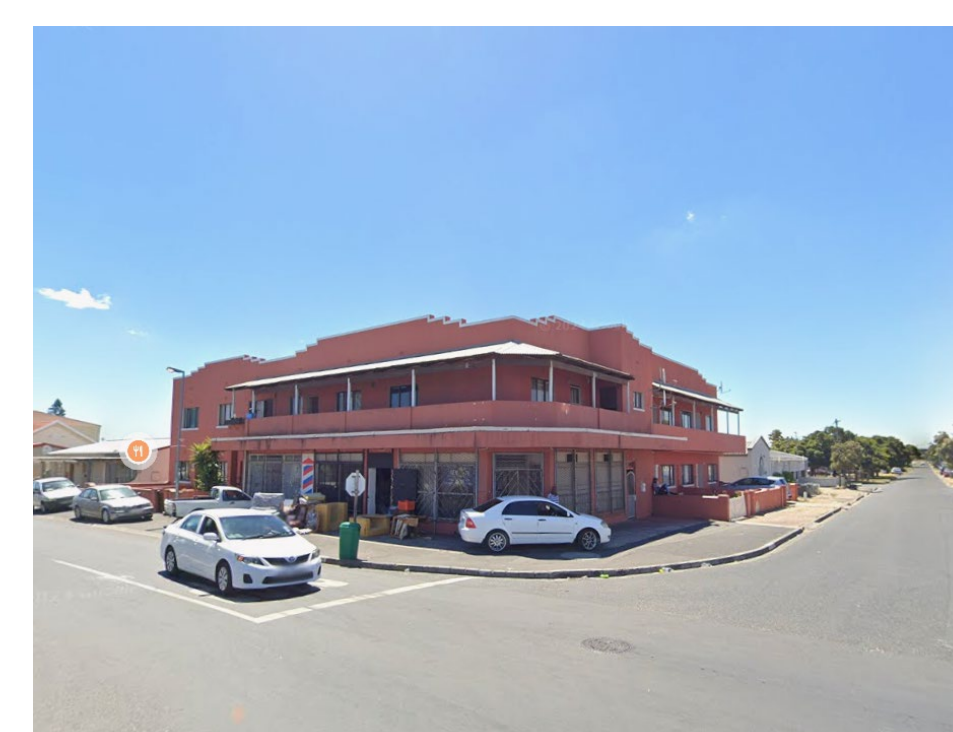
FIGURE 15: Existing Development along Bunney Street and 5 th Avenue
