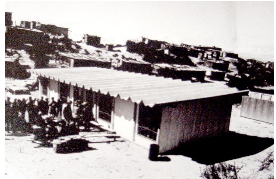
Photograph 4. Sizamile School, Crossroads (J. Cole Collection)
