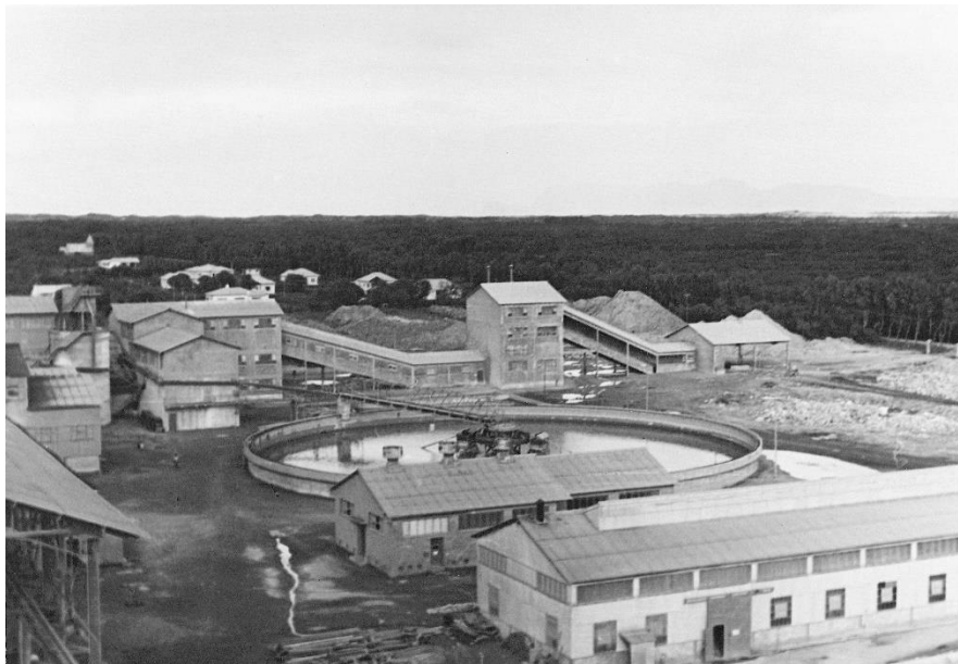
Photograph 2. The Cement Factory on Neu Eisleben Road in the late 1940s or early 1950s. The Neu Eisleben church is visible at top left (courtesy E. Wessels)
