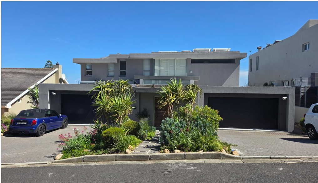
The Ronald Road street elevation of Erf 1003
