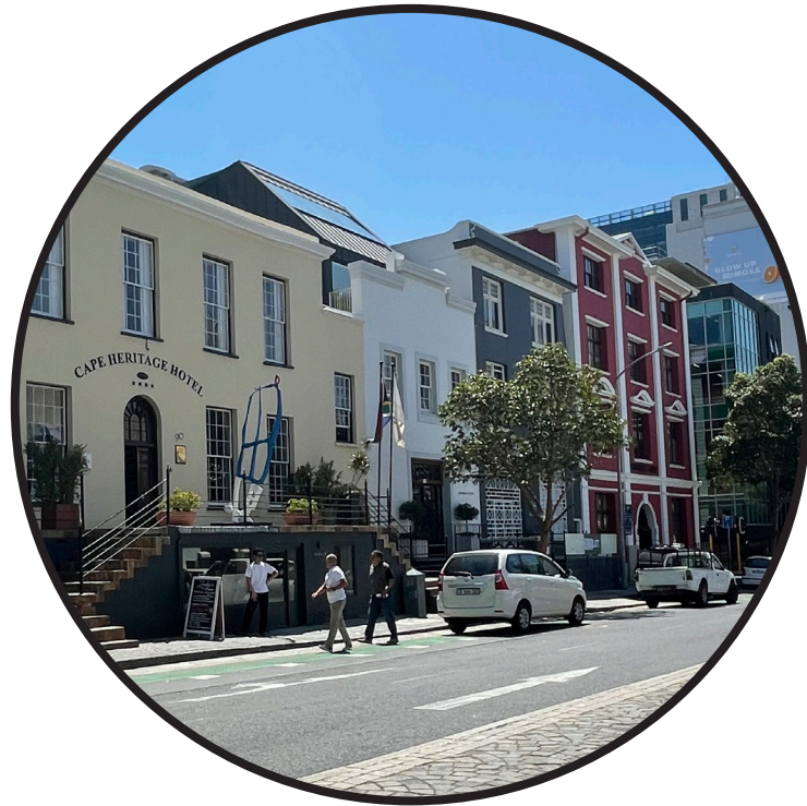
Sensitive addition behind a parapet
