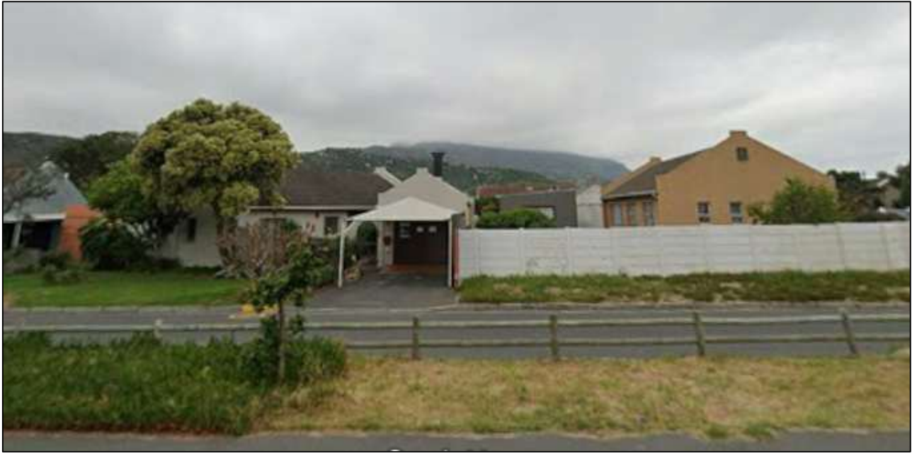
Figure 11: View of the existing dwelling from OU Kaapse weg. The fact that the proposal is limited to the existing development envelope and the new height of 4.891m of the gable not impacting the viewshed towards the mountain.
