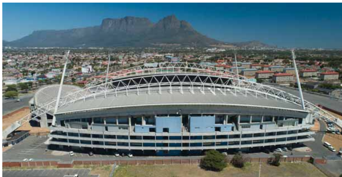
Stadium spruce-up: One of the City's capital projects in the central metro is the upgrade of Athlone stadium. Other projects include housing, road rehabilitation, development of MyCiTi routes, and upgrades to electrical infrastructure.
