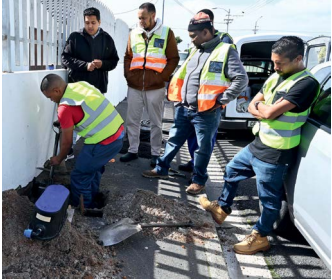
Getting stuck in: Mayoral Committee member for Water and Sanitation Cllr Zahid Badroodien (in the black jacket) with a team on-site in Athlone carrying out a water meter replacement.
