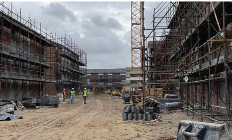
Going up: The Bothasig Gardens Phase 2 project is progressing well and expected to be completed later this year, providing social housing opportunities to 314 beneficiaries.
