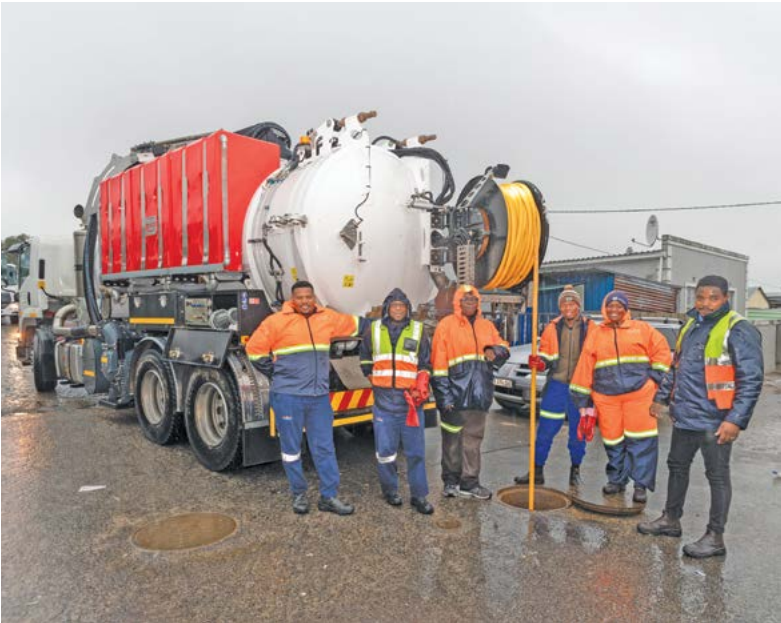
Pricey and preventable: The City's teams have their hands full keeping the sewer system in Dunoon clear of objects that do not belong there. Abuse of the sewer system is consuming far too much of the City's time and taxpayers' money.
