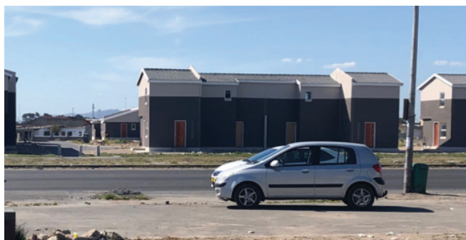
PHOTO 2. MAU MAU HOUSING DEVELOPMENT: EXAMPLE OF CURRENT LOW DENSITY 37 UNITS/HA
