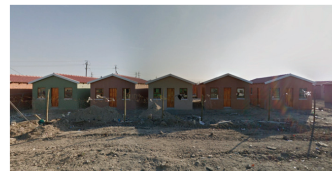
PHOTO 4. CROSSROADS HOUSING DEVELOPMENT: EXAMPLE OF MEDIUM DENSITY 67 UNITS/HA
