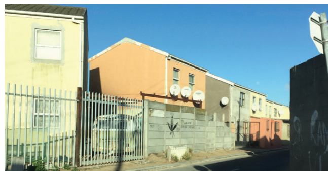
PHOTO 3. STOCK ROAD HOUSING- PHASE 1: EXAMPLE OF HIGH DENSITY
