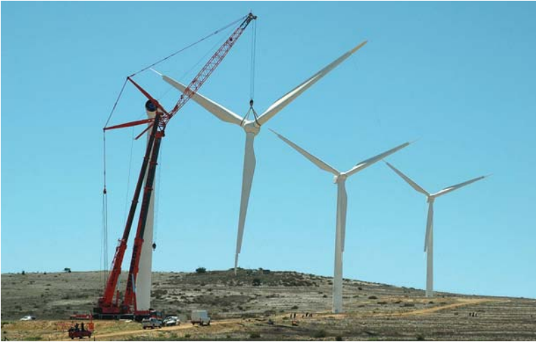
A green industry hub: The Atlantis special economic zone has attracted renewable-energy manufacturing, such as towers for wind farms.
