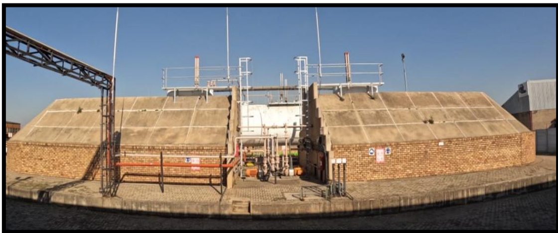
Fig. 7: Example of semi-buried tank design
