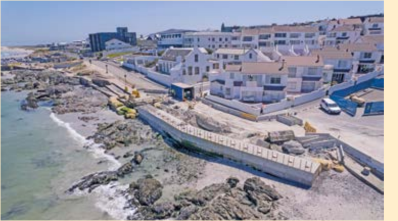
Willing the wall into existence: The project to reconstruct the Small Bay seawall, repair surrounding roads and re-route the old sewer line landward is on schedule for completion by September. Work, which started in early 2023, has been challenging, given the small footprint of the project area.
