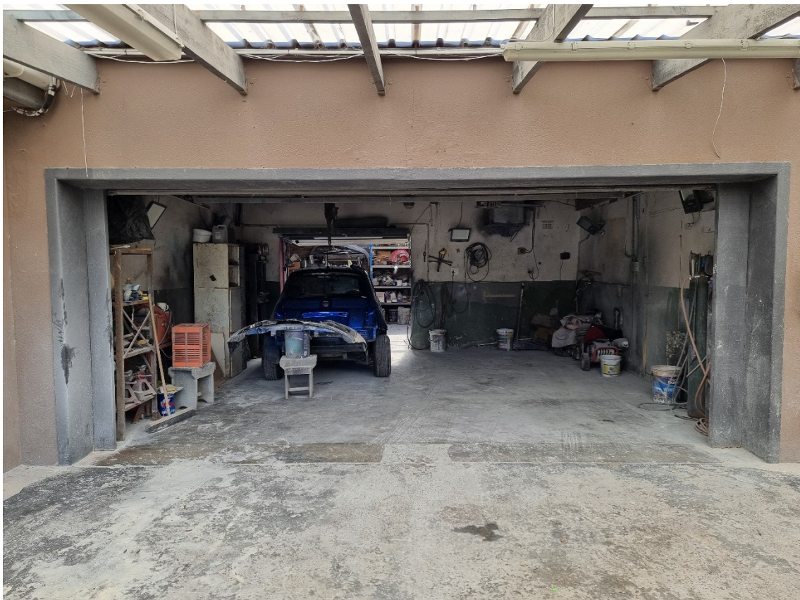
Figure 8: Image 02- Taken within the property facing the Spray booth.
