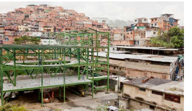
PHOTOGRAPH 12. MEDELLIN, COLUMBIA: MULTI STORY GYM- A CREATIVE SOLUTION TO PROVIDE RECREATION FACILITIES IN A LOCATION WITH SPACE CONSTRAINTS
