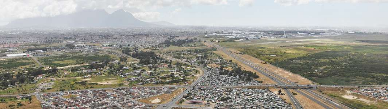
PHOTOGRAPH 5. AERIAL VIEW OF THE POA, SHOWING ITS PROXIMITY TO THE AIRPORT
