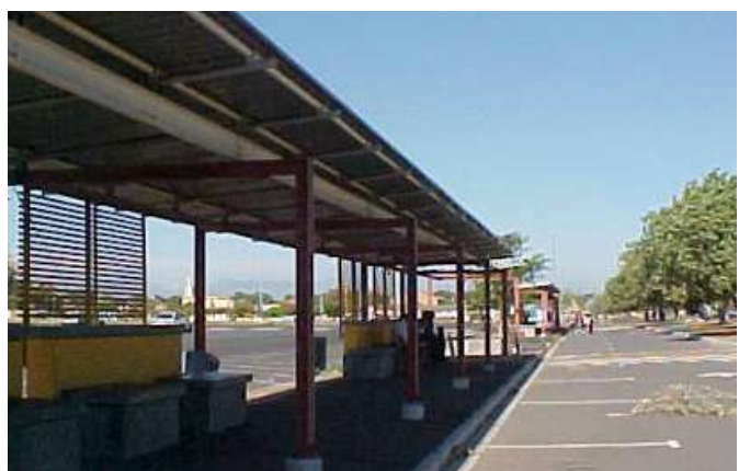
PHOTOGRAPH 14. ATHLONE STADIUM, KLIPFONTEIN ROAD
