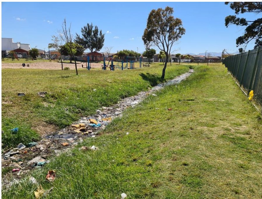
Figure 2.13: Illegal dumping in a stormwater swale
