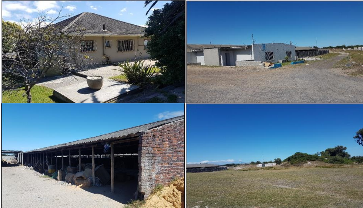
Figure 4b: Site Photos – Farm 790
