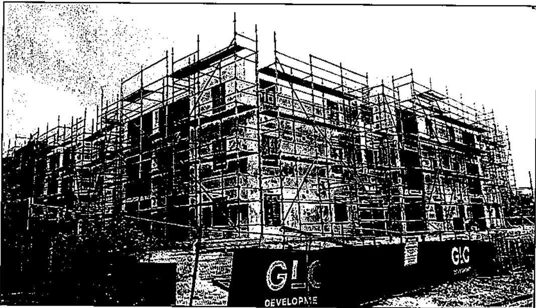
Figure 13 – The three-storey residential development on Erf 17360, currently under construction.
