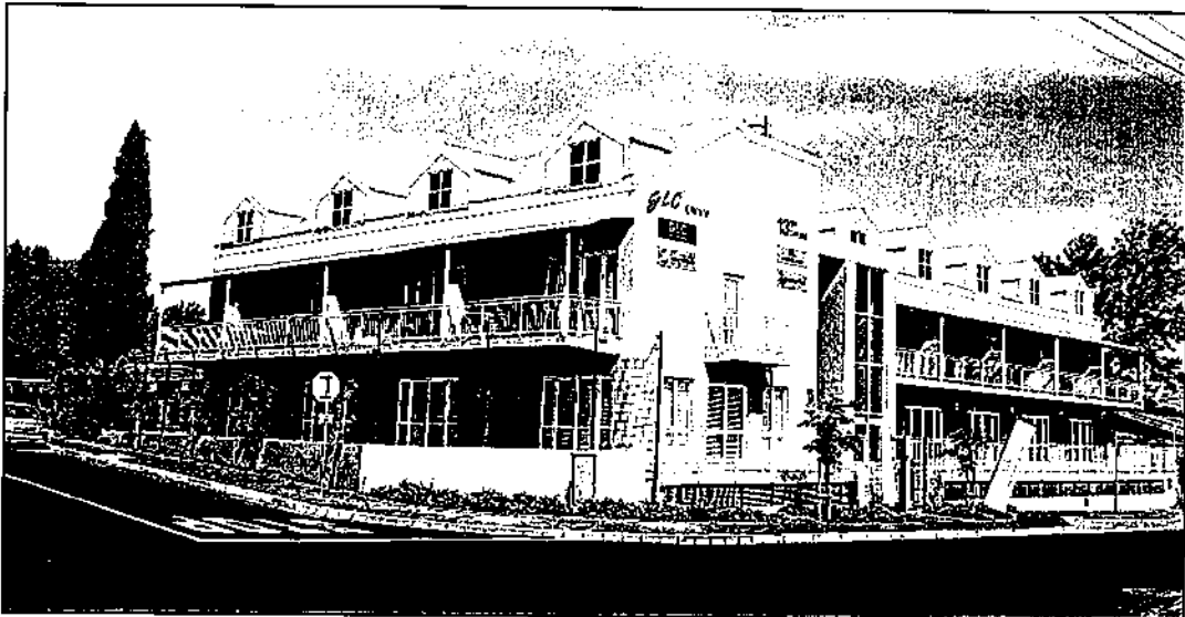
Figure 14 – The existing three-storey commercial development on Erf 1657, Durbanville
