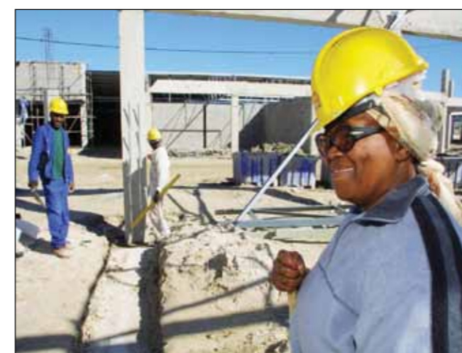
Construction of the Khayelitsha Centre.
