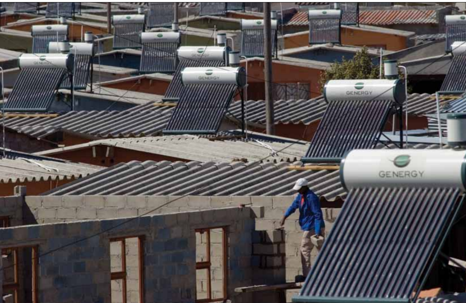
Solar water heaters in the Kuyasa Housing project.
