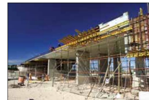
Khayelitsha railway extension project under construction.
