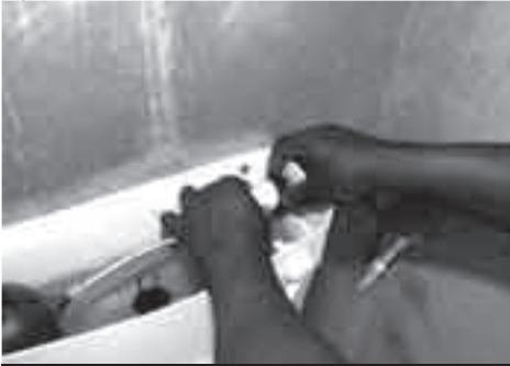
Replacing a float valve in a toilet cistern
