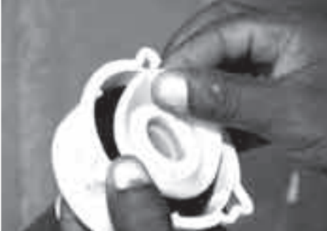
Fitting a new flush valve washer
