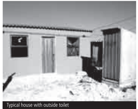
Typical house with outside toilet
