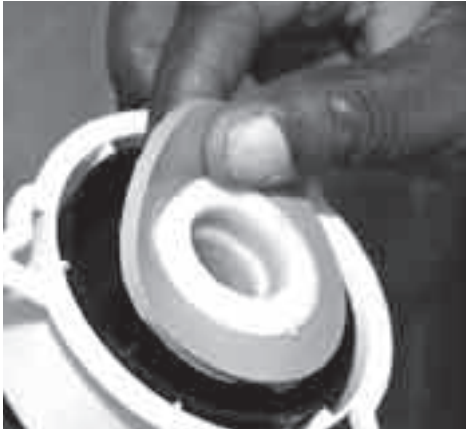
Removing a flush valve washer
