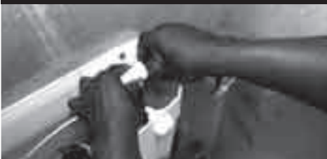
Replacing a float valve on a toilet cistern
