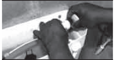
Replacing a float valve on a toilet cistern
