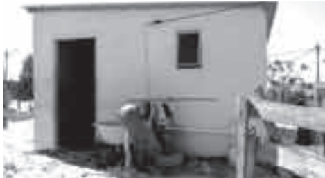
Typical house with inside toilet
