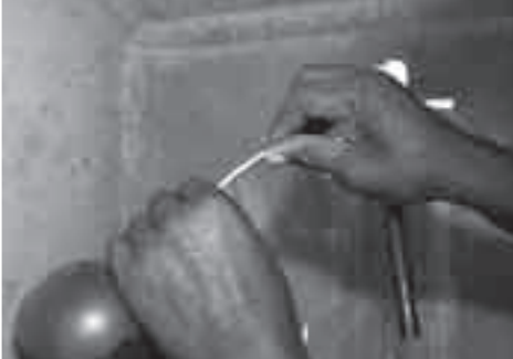
Adjusting the float arm
