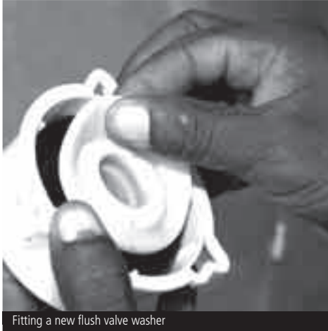
Removing a flush valve washer
