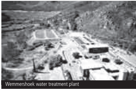
Wemmershoek water treatment plant
