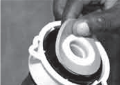
Removing a flush valve washer
