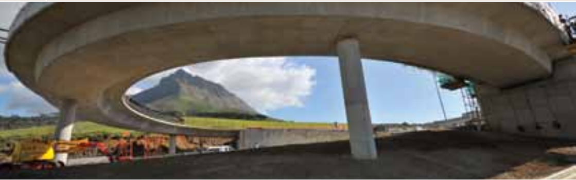
Construction work at Hospital Bend
