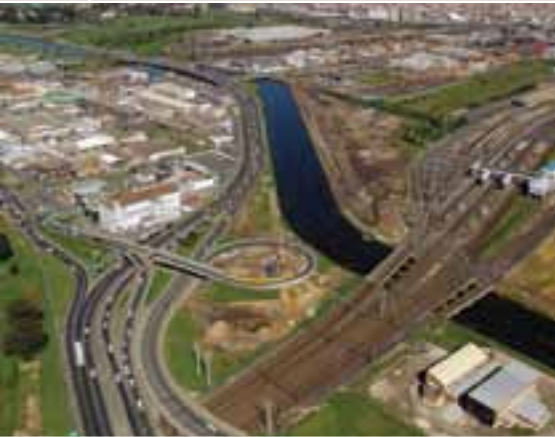
Koeberg interchange under construction
