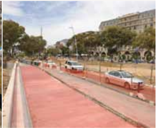
Bus-based IRT system under construction
