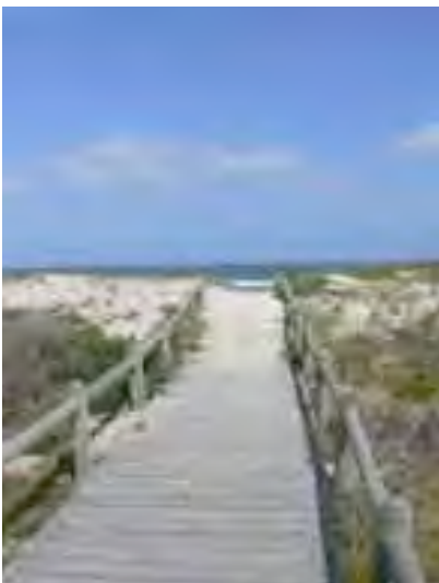
Rigid boardwalk in good physical condition, but covered with sand at Blaauwberg.
