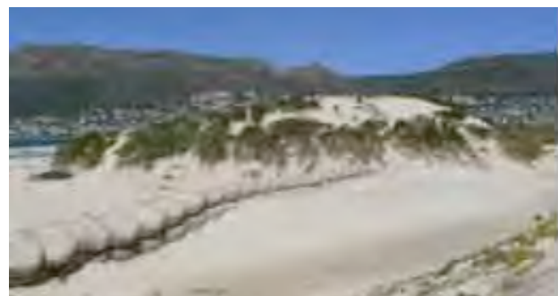
Sand bag type gabions are used to stabilise dunes at Clovelly. Wind-blown sand is a problem here as it affects the nearby railway.
