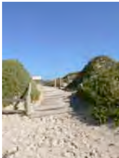
Boardwalk with broken fences at Fish Hoek. These boardwalks are chained and can be lifted as sand height increases, unlike the adjacent Blaauwberg boardwalk which is constructed like a bridge.
