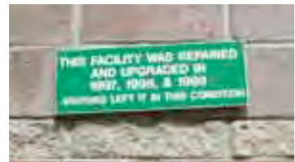
A sign at Silwerstroom Strand suggests that visitors to the area have a serious lack of respect for public property.
